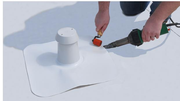
2. Install Two-Way Air Vents between fastener rows and at high points of roof area. Two-Way Air Vents must not be installed within 7 feet of the building edge. Never install Two-Way Air Vents in low, or drainage areas.
